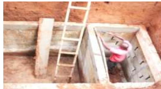
Fig. 17: Construction of the Septic tank / Soak-away pit
