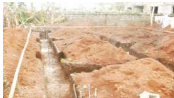
Fig. 16: The casting of the foundation footing
