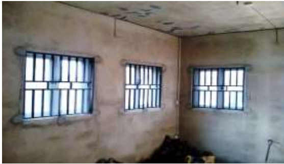
Fig. 20: Finishing of the interior spaces
