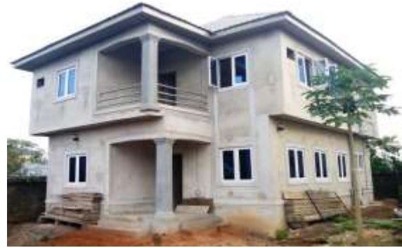
Fig. 21: Project under defects liability period
