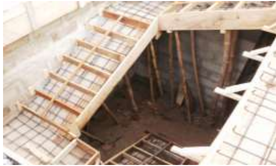
Fig. 19: Construction of the Stair case
