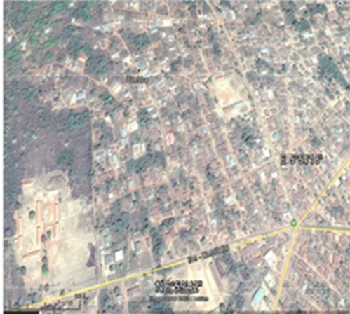
Fig 1: Aerial View of Uzebba Town (Source Google Earth)
