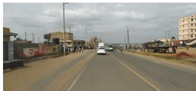
Scene 29 (Predominantly built-up roadsides with highrise buildings, Building material lying on the roadside, Unprogrammed parking, unpaved and dusty surface, Concrete electricity poles, Electricity lines, Moving vehicles, Pedestrians on the roadsides, Marked lanes, Undefined road shoulders, Abandoned truck bed on the roadside, Concrete open drainage channel)
