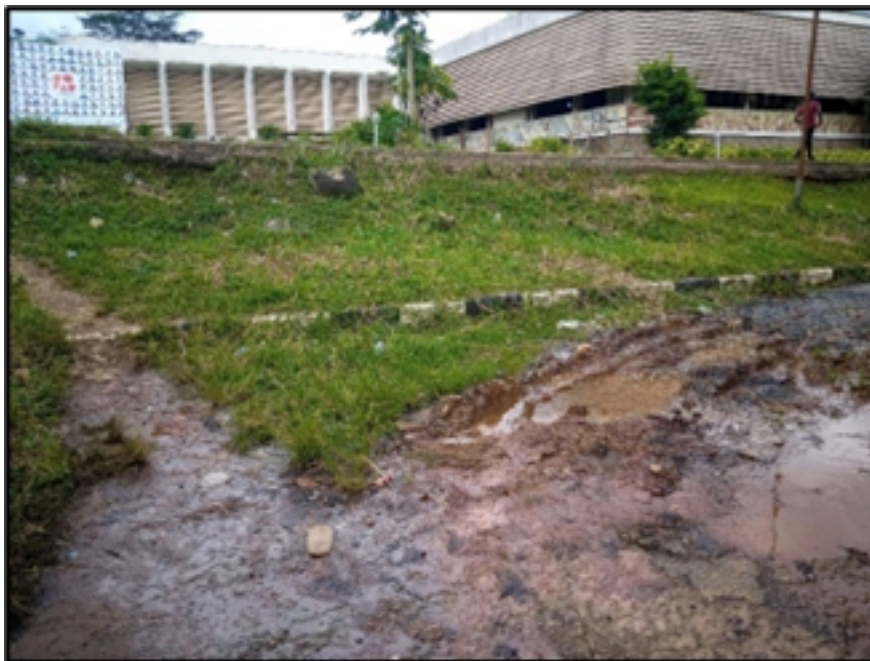
Figure 7: Groundwater seepage at the Department of Geology car park.
