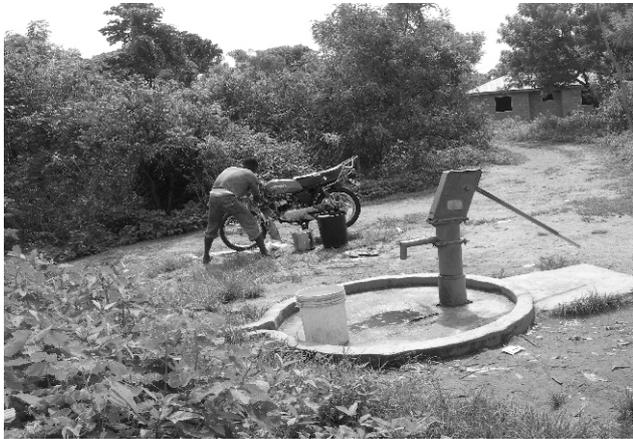
Figure 6a: Hand Pump Borehole as Source of Water Supply
