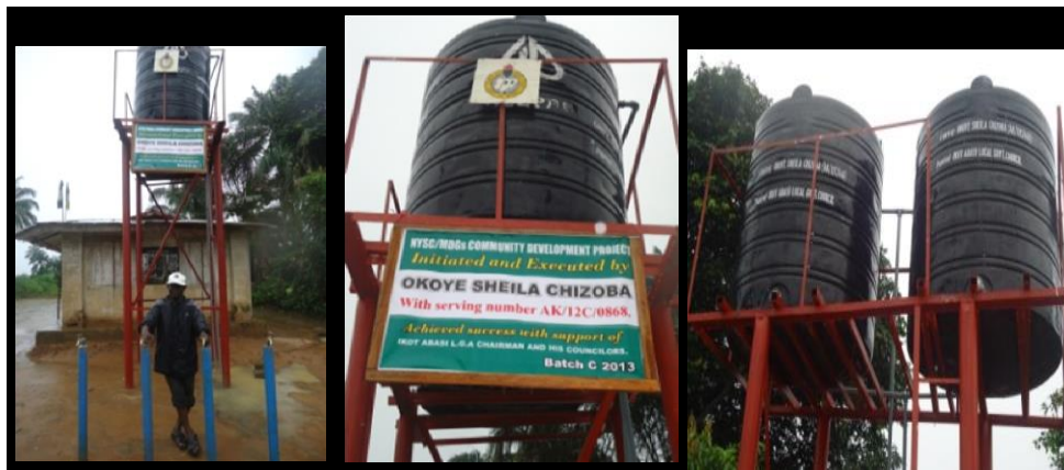
Fig 3: Front view of Overhead water storage at Ikot Abia Ndia villages Edemaya of Ikot Abasi L.G.A. Akwa Ibom State.
