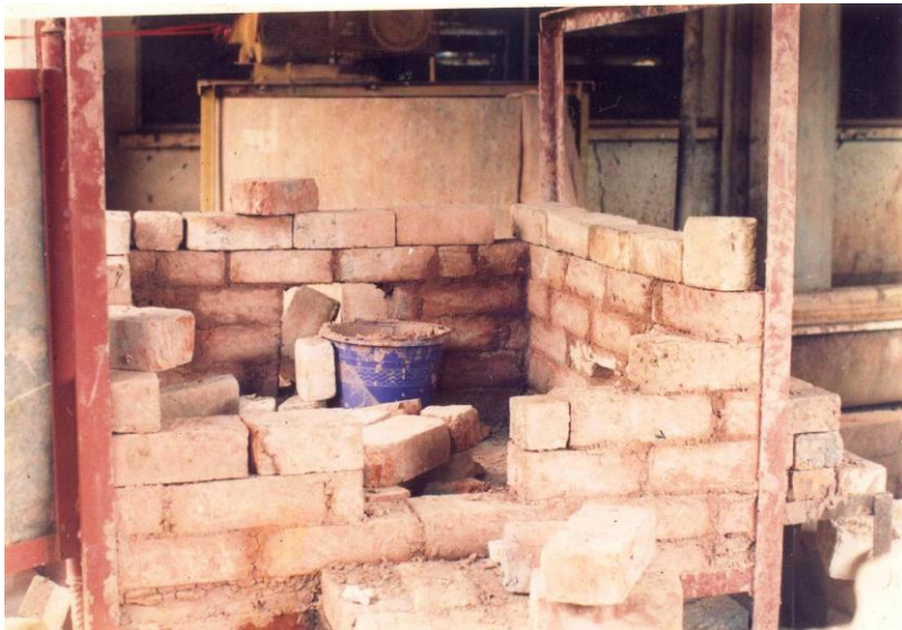
Fig. 5: Kiln building in progress
