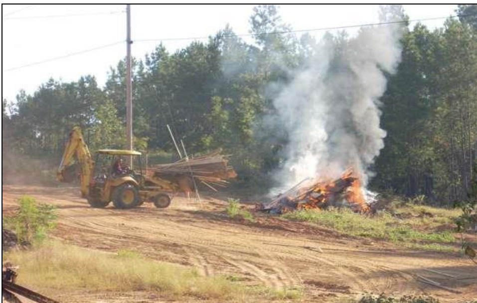
Figure 3: Burning of slabs near Forest Stand can Facilitate Forest Fire if done without Precautions
