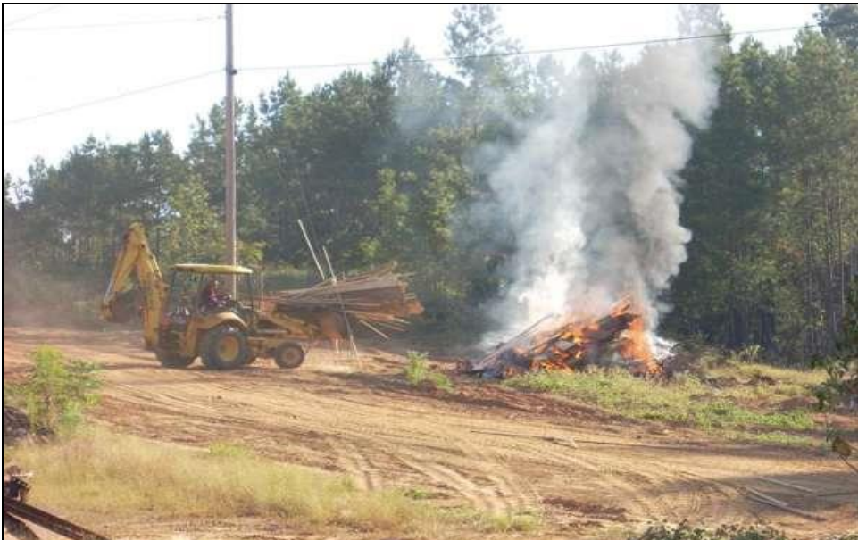
Figure 3: Burning of slabs near Forest Stand can Facilitate Forest Fire if done without Precautions
