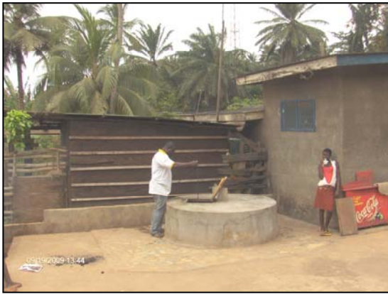
Fig. 5a Typical Open Top Hand Dug Well with Clean Surrounding
