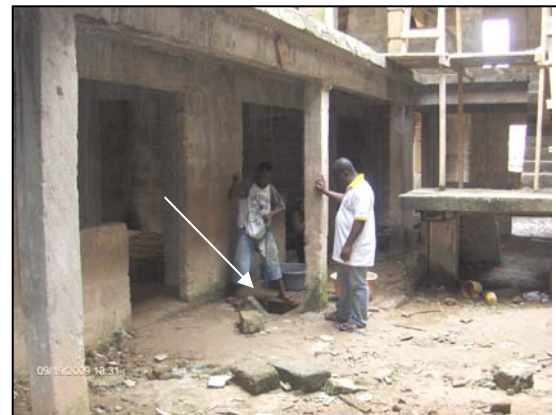
Fig. 5d Within the Compound of the house mentioned in Fig. 5c is a Well (arrowed)
