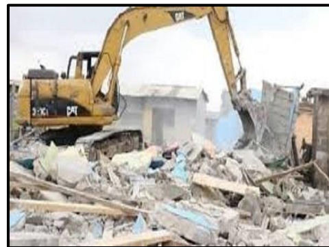
Fig. 3 Demolition Exercise at Frafraha
