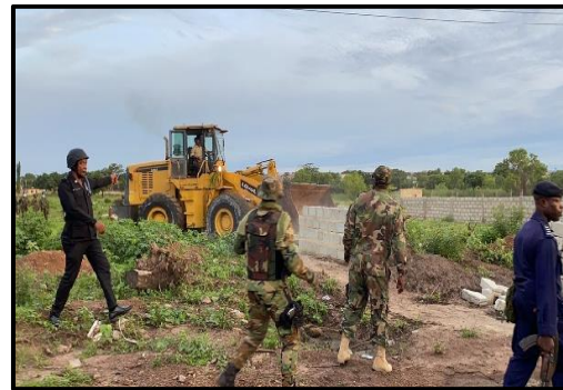
Fig. 2 Demolition Exercise at Frafraha
