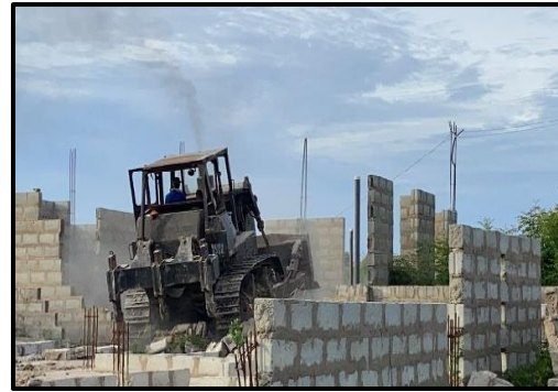
Fig. 1 Demolition Exercise at Frafraha
