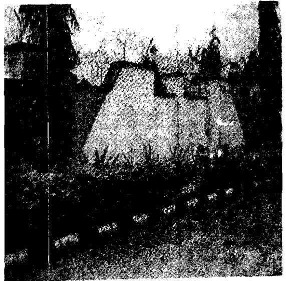
Figure 1: A solid fence wall in one of the housing estates with electrified barbed wire.
