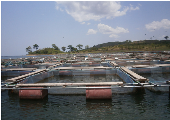
Fig. 4. Fish cage comprising galvanized pipes, metal drums and nylon nets
