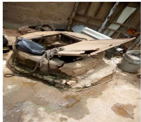
Plate 1: Well Rusted Metal Cover in Ikwa ward Source: Field work, 2019
