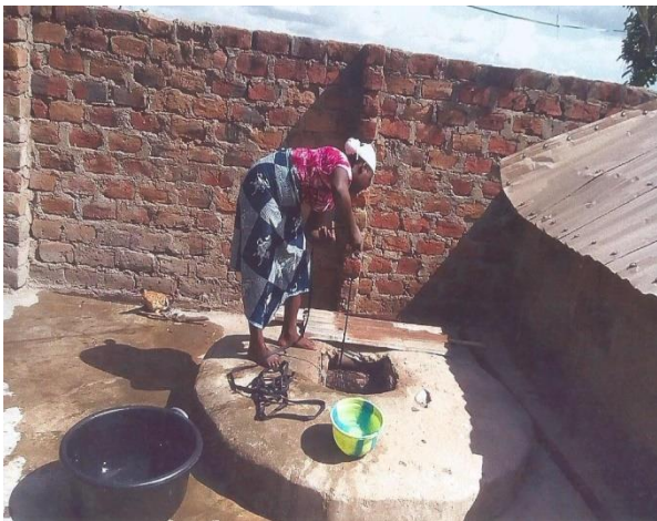
Plate 1: Well Without Cover in Ikwa ward Source: Field work, 2019
