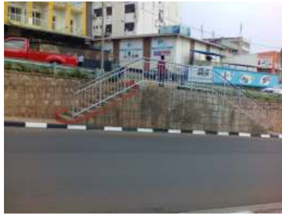
Figure 13: a stair case on KN1Rd built recently in 2019
