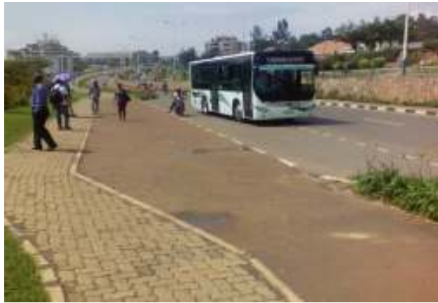
Figure 12: Bus stop without pedestrian shelter on KN501St
