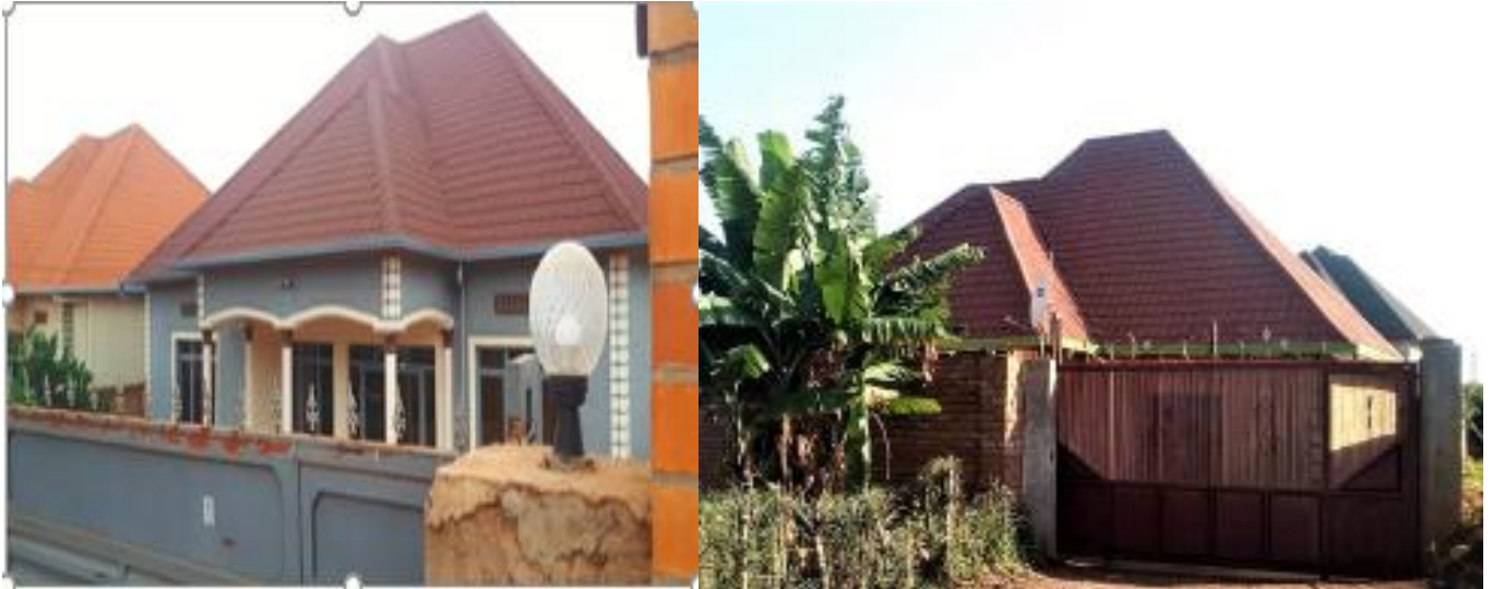
Plate 4: Modern steep roof pitch
