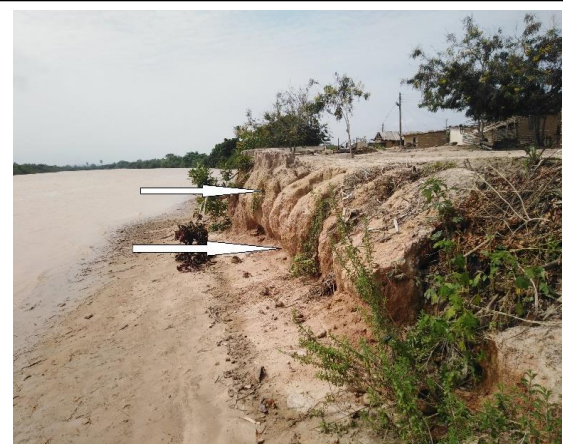
Figure 4b: Riverbank erosion at Bosomdo Source: Field survey, 2019
