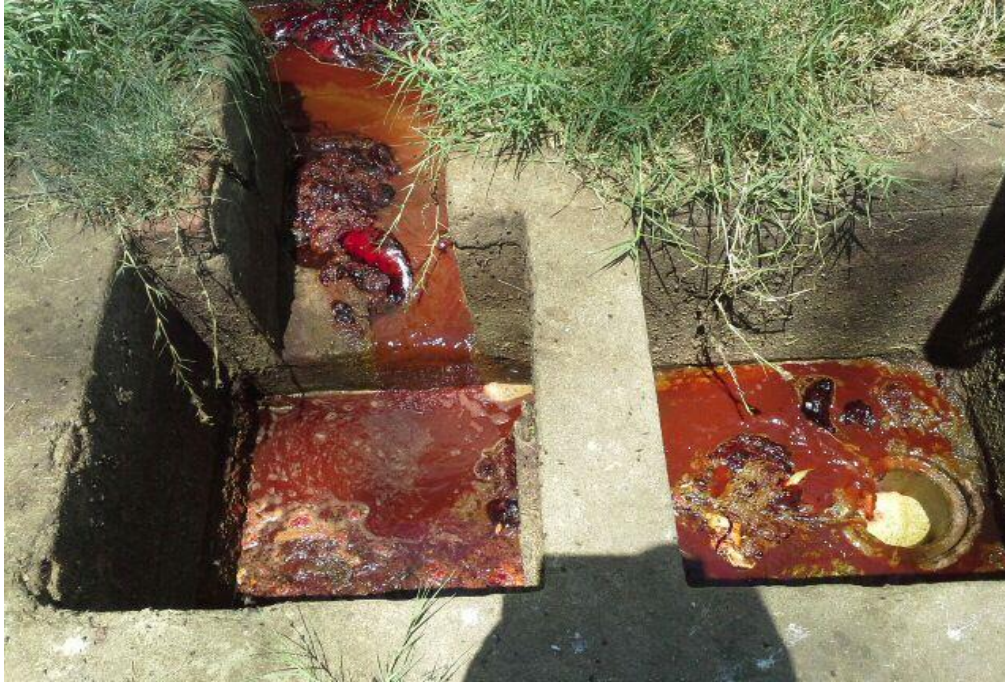
Plate 2: Slaughter waste being discharged direct into the sewer system
