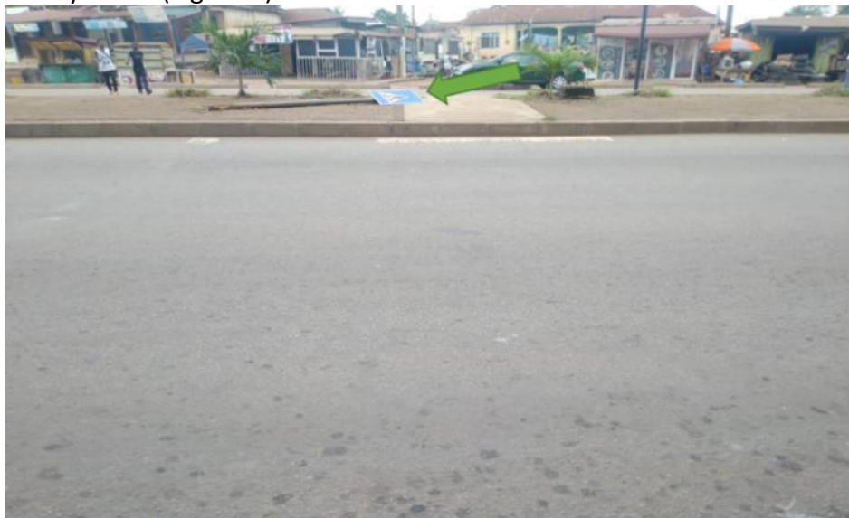
Figure 14: Signage requiring maintenance attention
