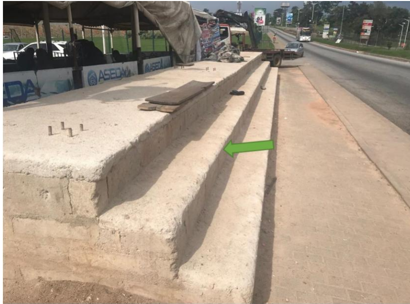
Figure 24: A rest stop under construction at KNUST Junction with steps
