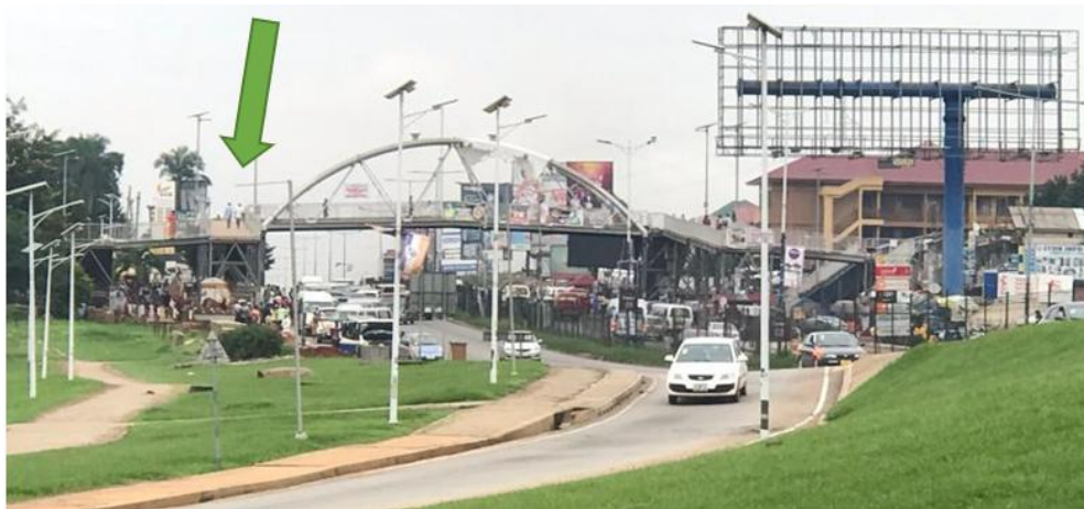
Figure 17: Footbridge at KNUST Junction
