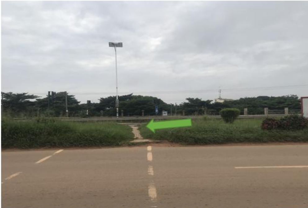
Figure 9: Lack of kerb ramp at crossing at AAMUSTED
