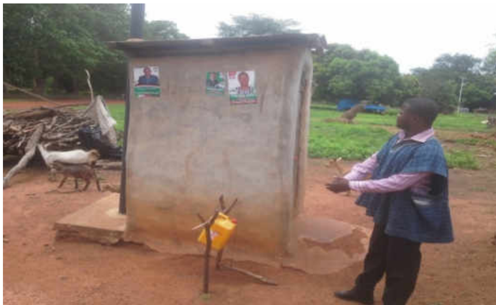
Figure 2: Pit latrine and tippy tap facility in Mognori Community
