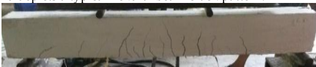
Fig. 15. Typical crack pattern of flexural beam specimen (Ansa & Mohan, 2015)
