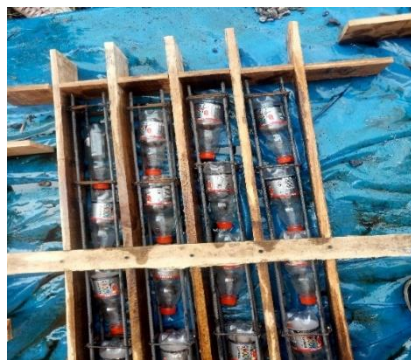
Fig. 3: PET bottles arranged in the beam mould
