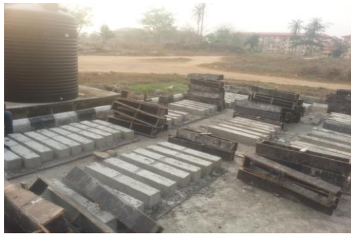
Fig. 5: Casting and demolding of beam specimens
