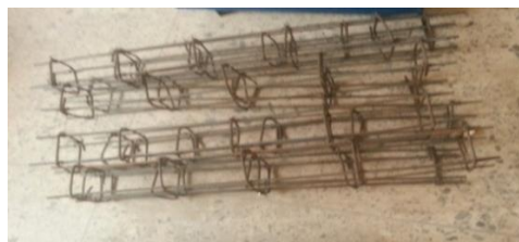
Fig. 2: Steel reinforcement with links in beams
