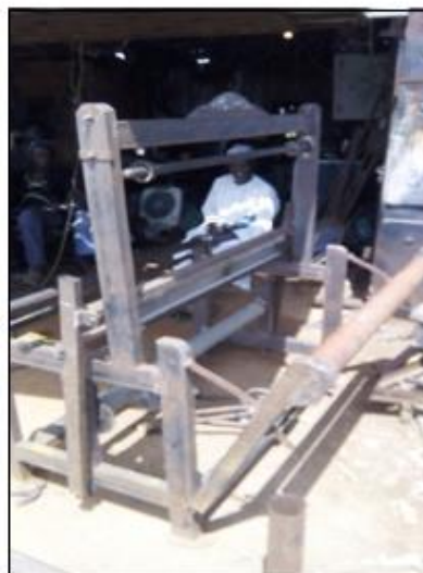
Plate 4: Constructed Steel frame
