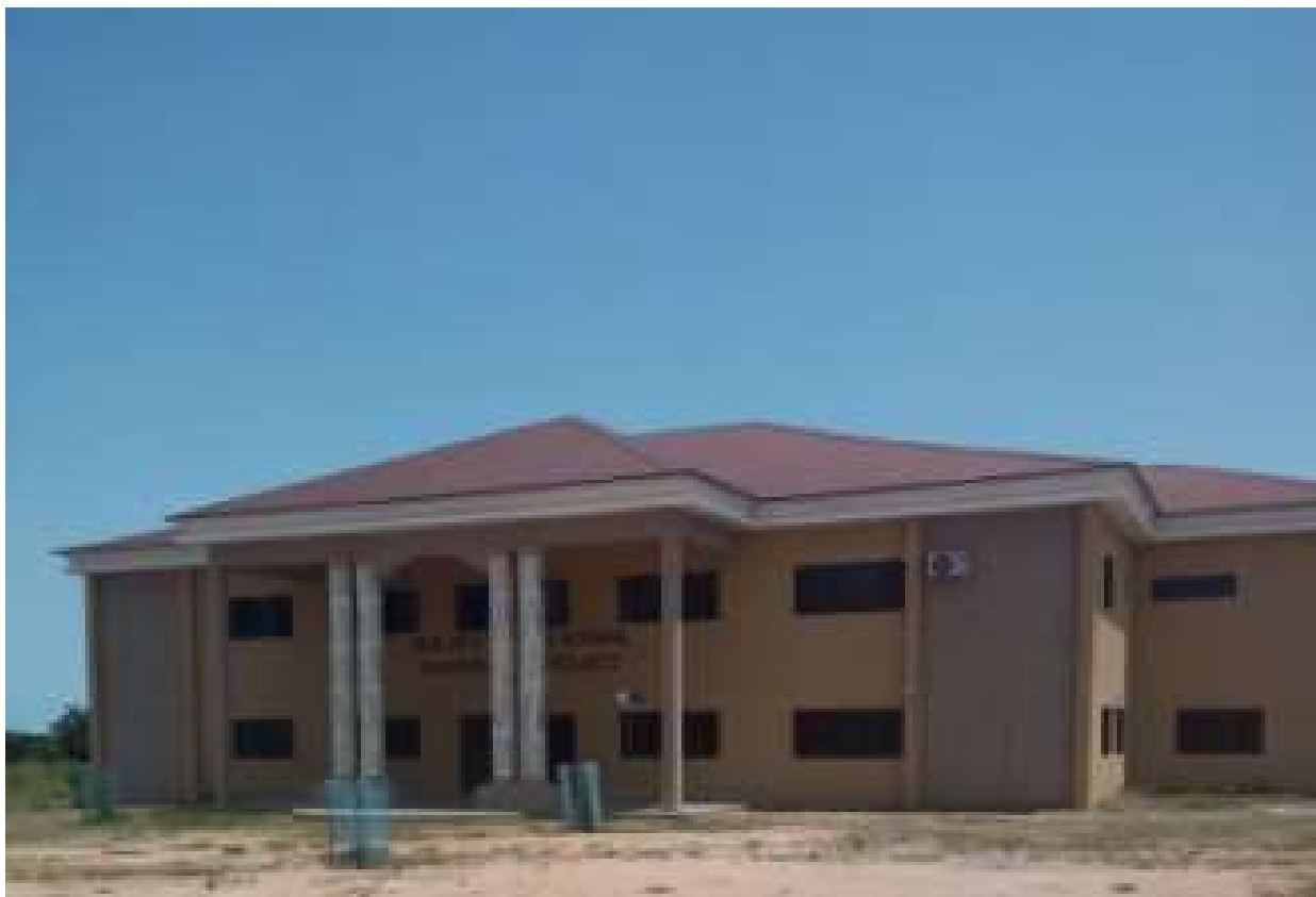
Figure 1: The School Environmental Sciences prototype building.
