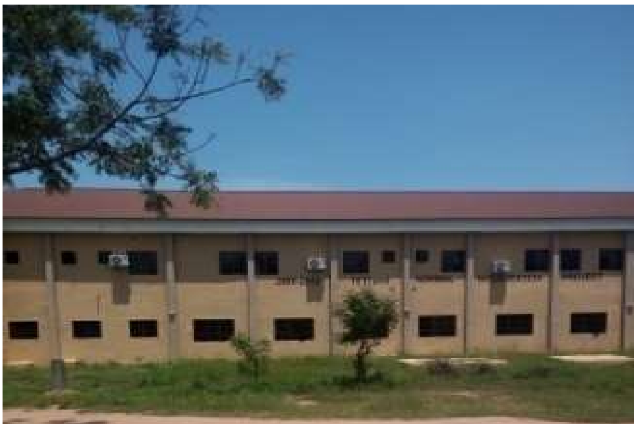
Figure 2: The SES prototype building (South Elevation)
