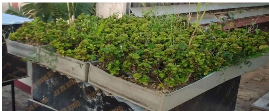
Plate 8: The observed green roof blends on site
