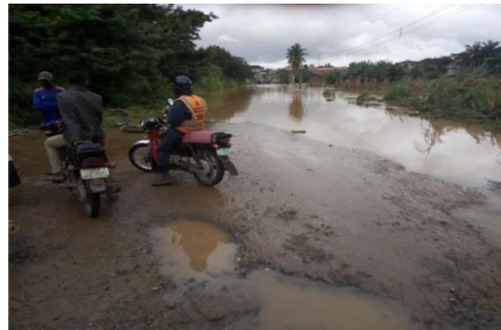
Plate 1.5: Storm runoff as flood along Ede Road in Ile-Ife
