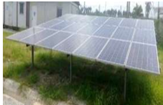
Figure 2.4: Experimental Setup at the Location: 2.4 kWp Solar PV array
