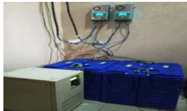
Figure 2.5: Experimental Setup at the Location: Inverting Unit, Storage Battery and Charge Controller Assembly
