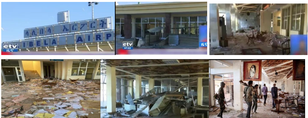
Figure.18. Damaged Infrastructure (Lalibela International Air Port) by TPLF
