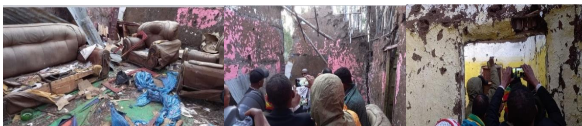
Figure. 21.Privet home, Hotels Damaged by TPLF @ Gayinte-Amhara
