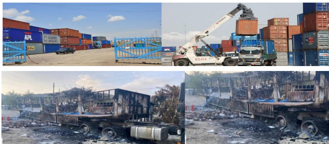
Figure 29. Damaged Infrastructure by TPLF Terrorist Group @Kombolcha-Dry Port-Amhara
