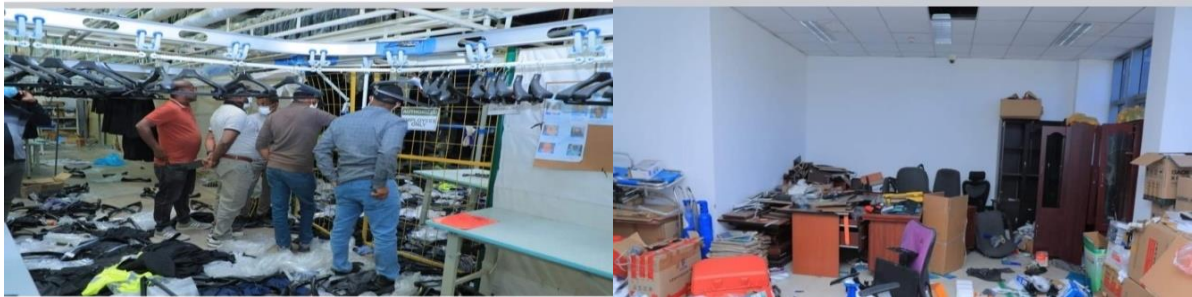
Figure.16. Damaged Infrastructure (Kombolcha Industrial Park) by TPLF
