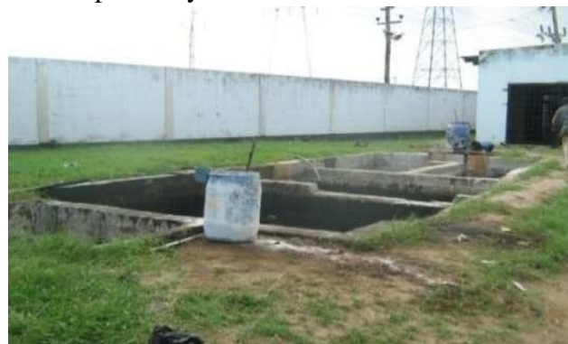
Plate 1b Waste Stabilization pond
