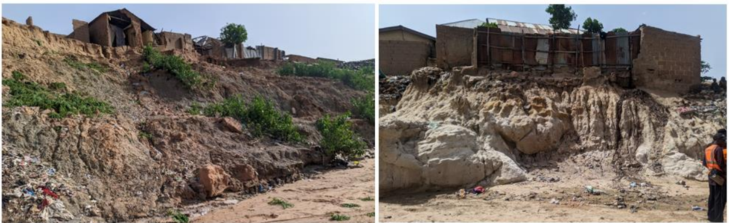
Fig. 10 Gully-induced slope failures in the moderately stable zones along Pantami Stream
