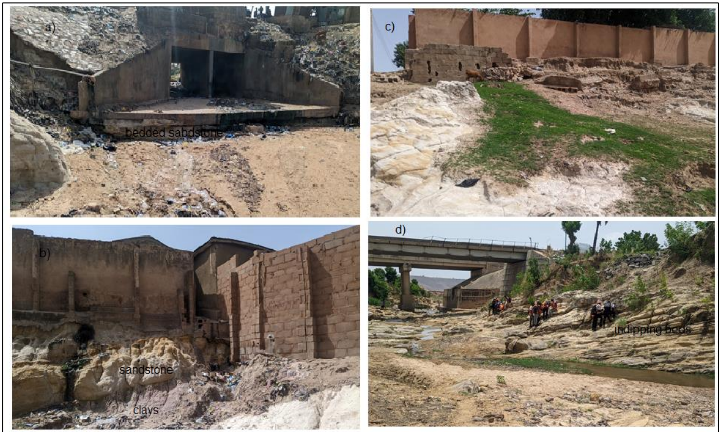
Fig. 9 (a) Unstable bridge founded on a bedded sandstone foundation, (b) Unstable buildings founded on sandstone with clay interlayer, (c) Stable building founded on massive sandstone, (d) Stable bridge resting on an inclined bed of Yolde formation along Doma Stream
