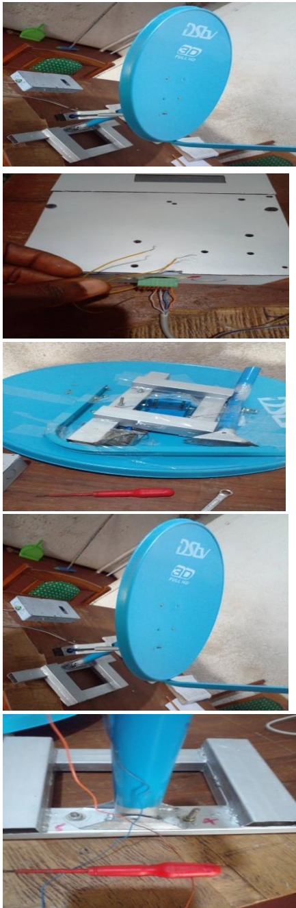
Figure 3.1: Installation process of the remote-control dish antenna
