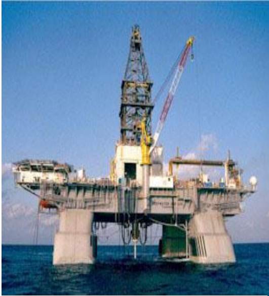
Fig.1 Deepwater Horizon prior to explosion Source: (WIKIPEDIA, 2011).
