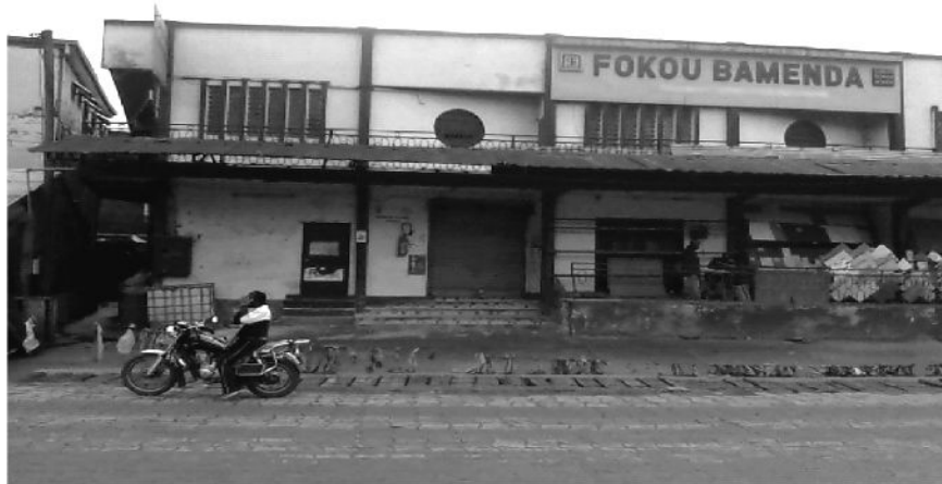
Image 6: Cinema Rota in Nkwen, closed in the early 2000, is now housing a building material shop of Cameroonian group Fokou. © Paul Animbom, august 20, 2017.
