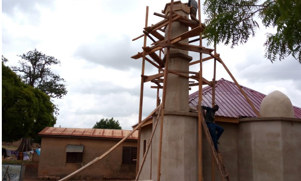
Figure 3: A mosque under construction using ‘modern’ building materials.
