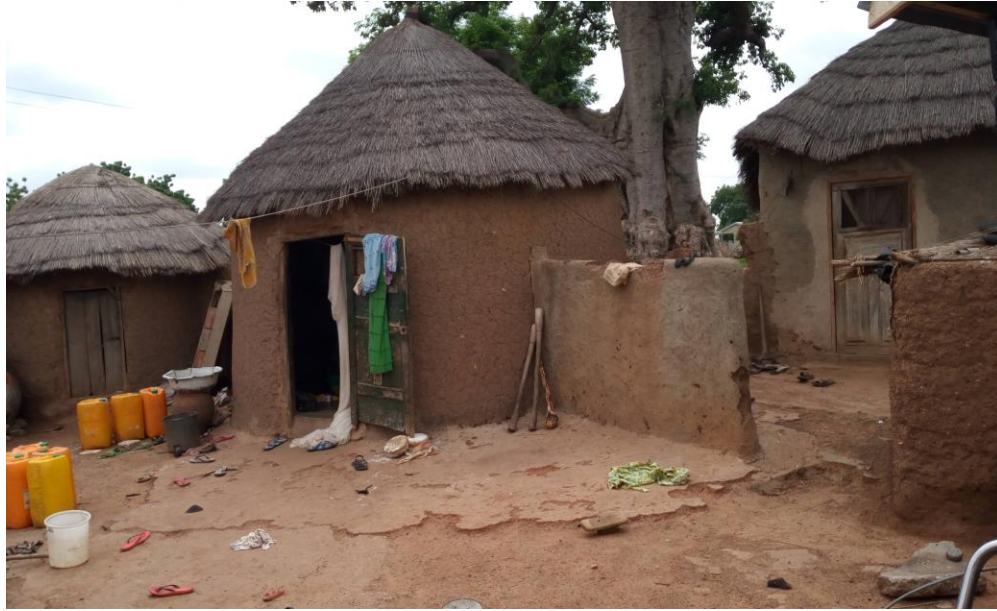
Figure 4: Family house depicting the traditional architecture of thatch roof, mud walls and round shape.
