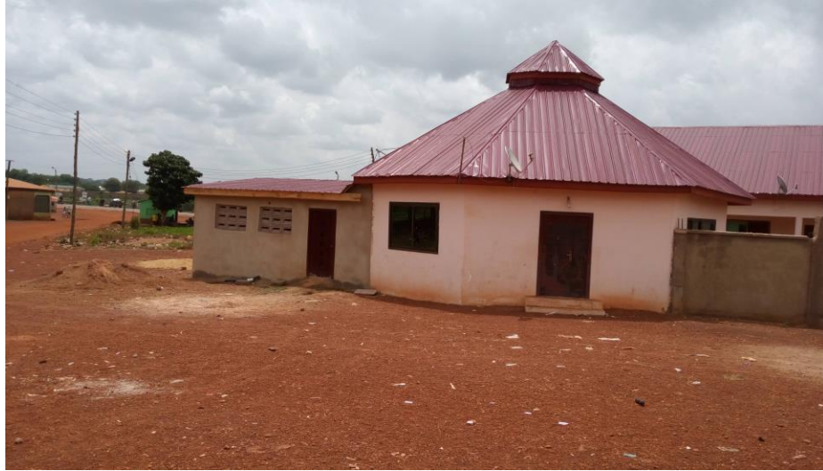
Figure 6: The Vittin chief's palace depicting a modern house. The walls are built with cement blocks and painted. It is roofed with metal sheets instead of thatch.
