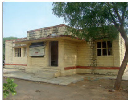
Fig. 4. The project was implemented in vacant staff quarters behind the community health centre in Gulbarga, Karnataka.
