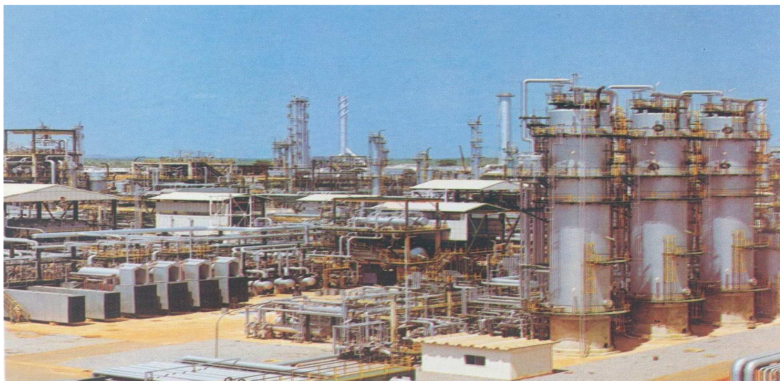
Figure1: Pictorial View of KRPC Asphalt Blowing Unit (Adapted from KRPC Site)
