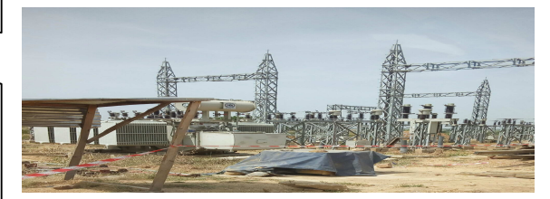
Site 'A' During Hydropower plant constructions in 2017
