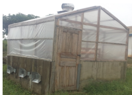
Figure 1b: Solar Tent Dryer
