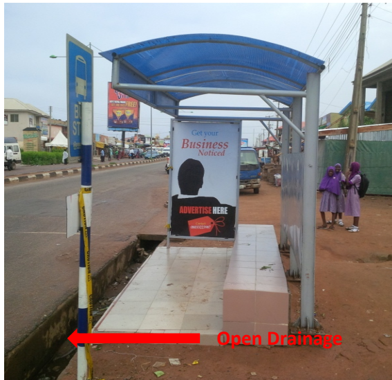
Figure 7(a): Simple bus stop shelter in Ilorin
