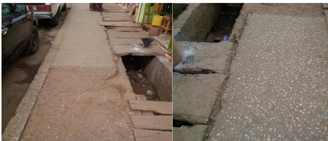
Figure 6: Sidewalks and drainage system along Murtala Moh'd Way
