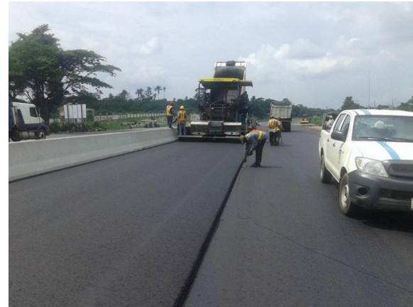
Figure 6. A View of the Lagos-Ibadan Expressway Project Source: https://www.nairaland.com/3234261/photos-on-going-rehabilitation-expansion-lagos-ibadan (Retrieved May 2024)
