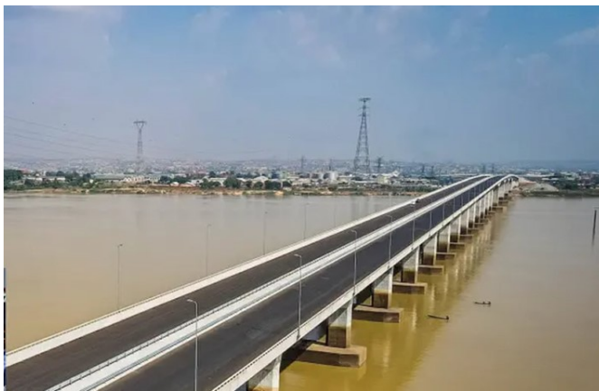
Figure 5. A View of the second Niger Bridge Source: https://punchng.com/second-niger-bridge-ready-for-commissioning-fg/ (Retrieved May 2024)
