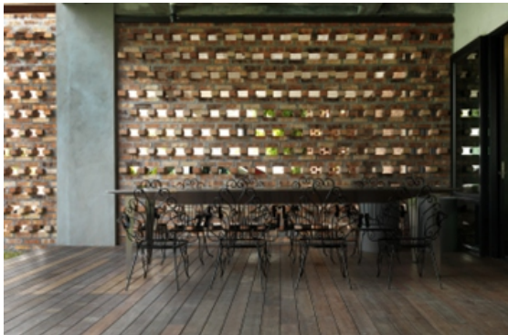
Figure 3: S11 house screen wall at outdoor dining Source: Archdaily.com, 2024
