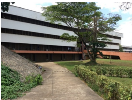
Figure 17: Use of horizontal concrete fins as shading device of the Hezekiah Oluwasanmi Library, Obafemi Awolowo University. Source: Researchers field work
