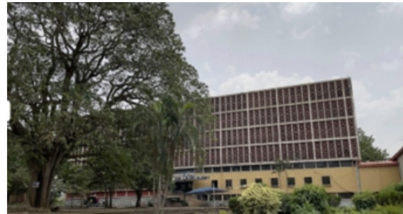
Figure 18: Use of Brise soleil as shading device of the Kenneth Dike Library University of Ibadan. Source: Researchers fieldwork
