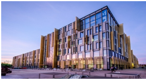
Figure 16: Use of vertical aluminium fins as shading device of University of Birmingham's Library. Source: Archi daily
