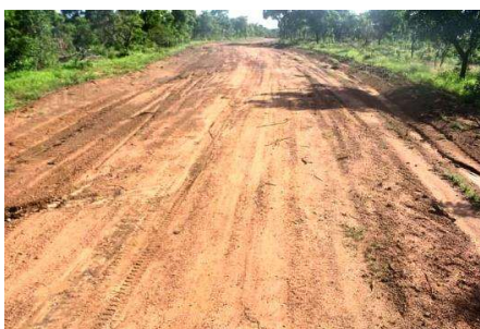
C: Newly Opened Road from Pina to Nitalu, Piina to Tanla
