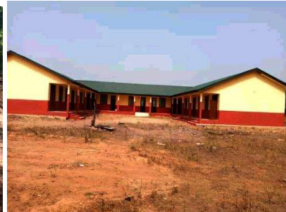
D: 6-Unit Classroom Block at Naabugujan
