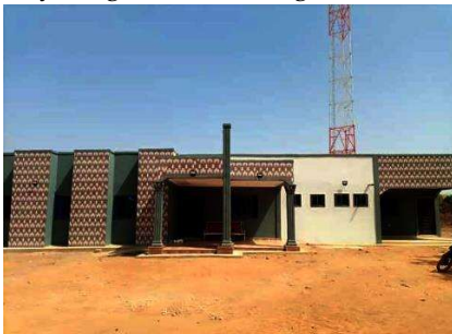
A: Chinnia MP's Office Complex with Ancillary Radio Station at Tumu.
