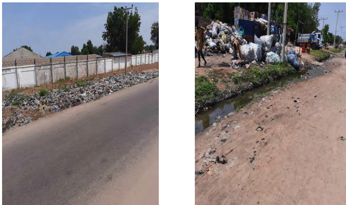
Figure 1: Images of waste dumps on road-sides ( left ) and blockage of storm drains ( right )
