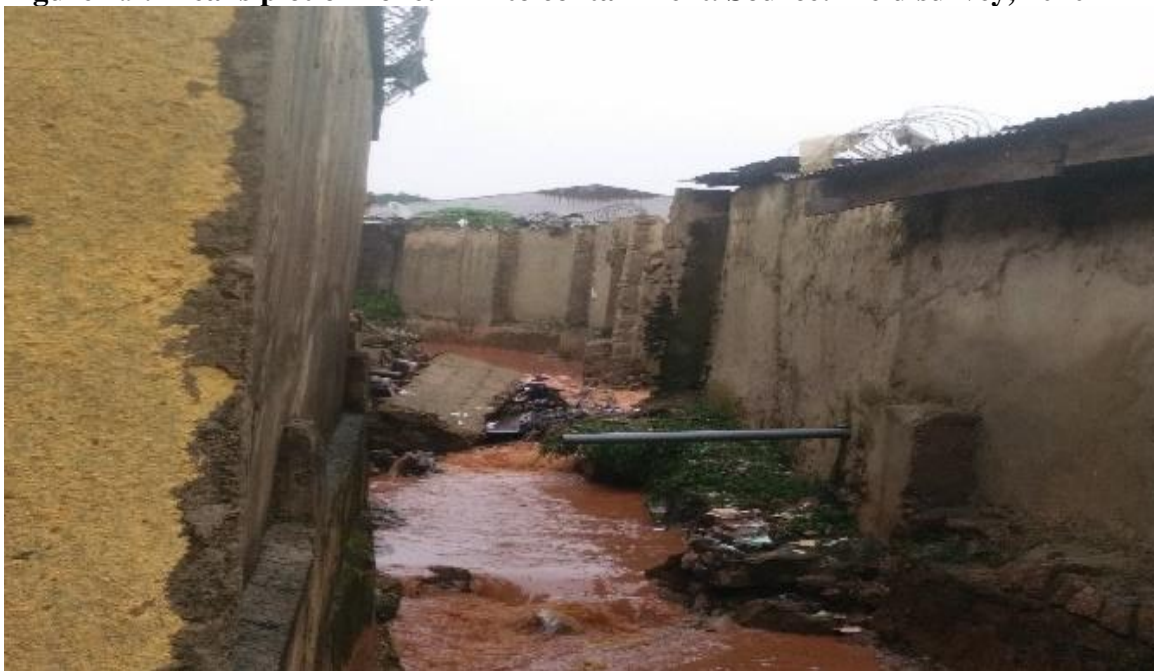
Plate 3: Toilet sewer directly linked to a stream in Kawo high-density. Source: Field survey, 2020
