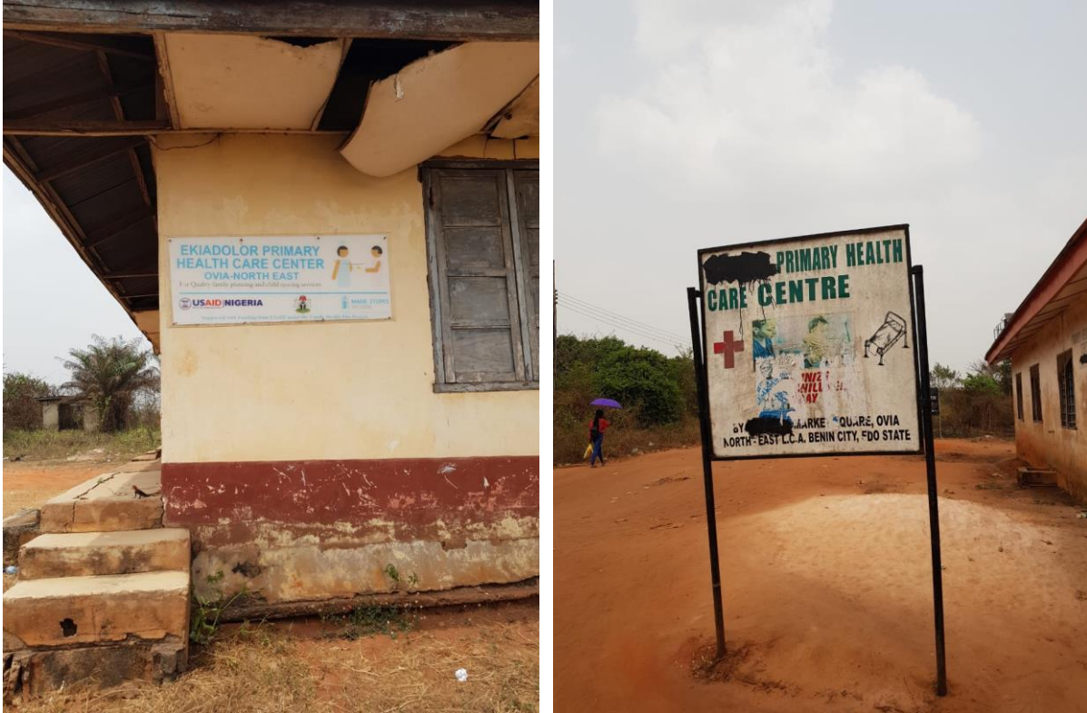
Figure 3: WASH facility in a PHC in Edo State, Nigeria (WHO 2019) 5
