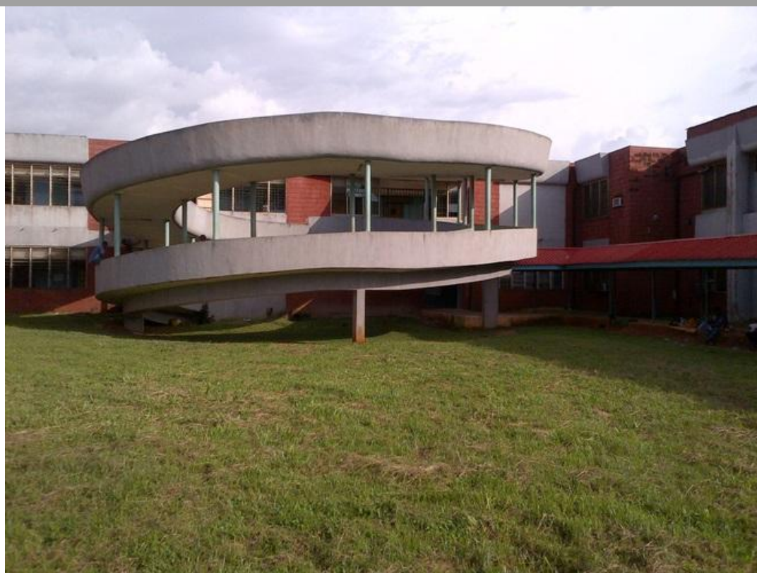
Figure 5 Ramp for conveying patients between floors of the complex.
