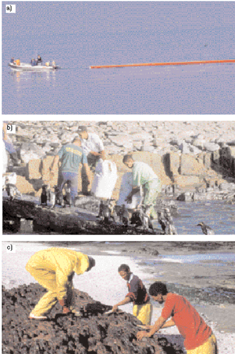
Fig. 3: A boom being deployed from the breakwater at Murrays Bay Harbour (a) and application of peat-based absorbents to rocks at (b) Robben Island and (c) Dassen Island
