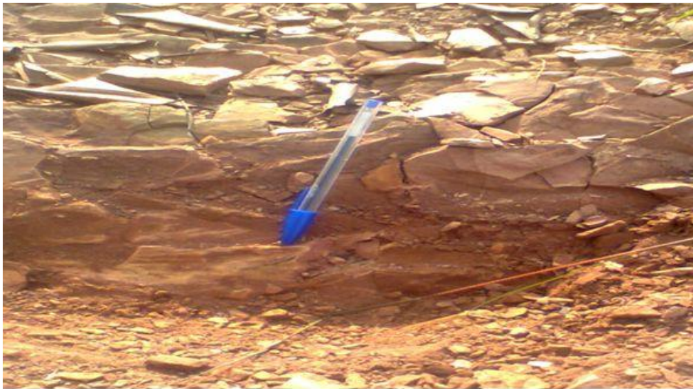
Figure 6. The joints in the brown shale unit.
